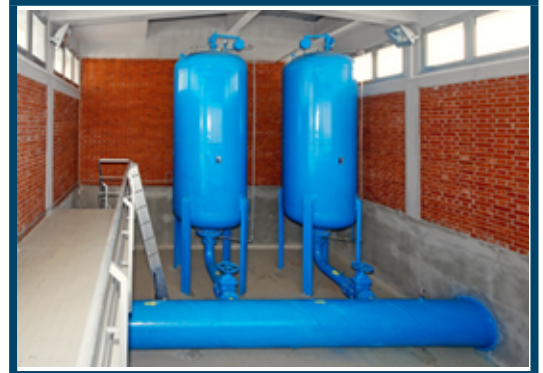
Figure 2 Two vertical air receivers
